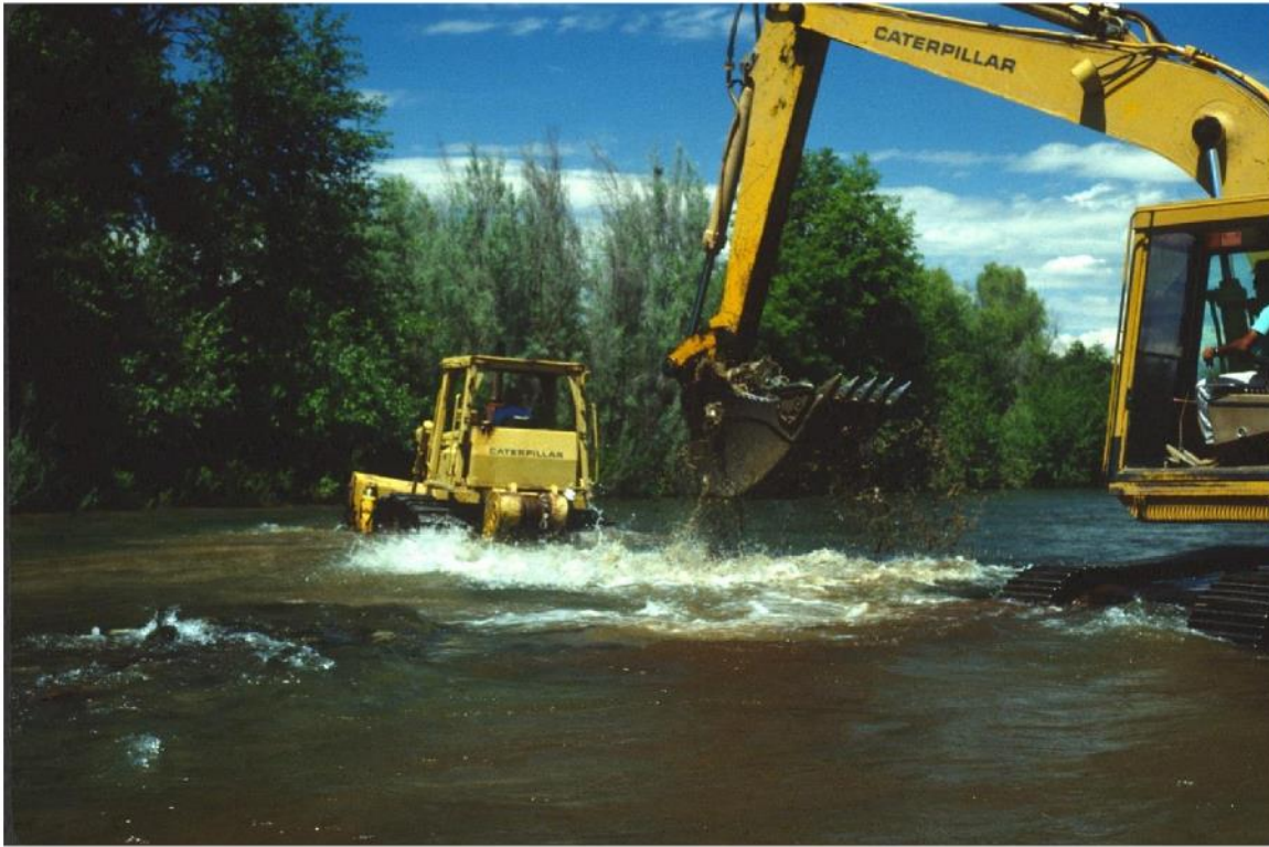
Gravel Cleaning Experiments using an excavator
